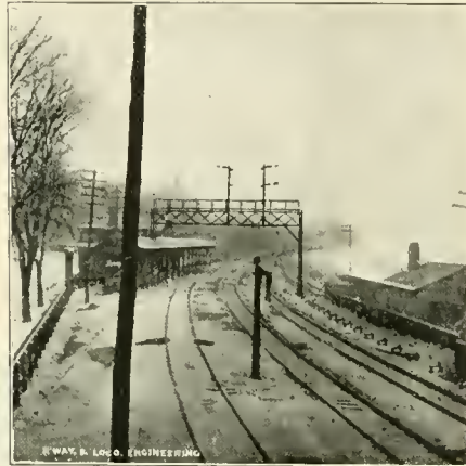
TYPICAL SIGNAL BRIDGE ON THE NEW YORK CENTRAL RAILROAD.
